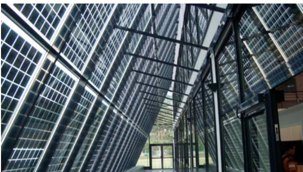
Figure 2: Inside the Building: The Corridor between the Photovoltaic Windowed Façade (Left) and the Robotics & Ambient Intelligence Area (Right)
