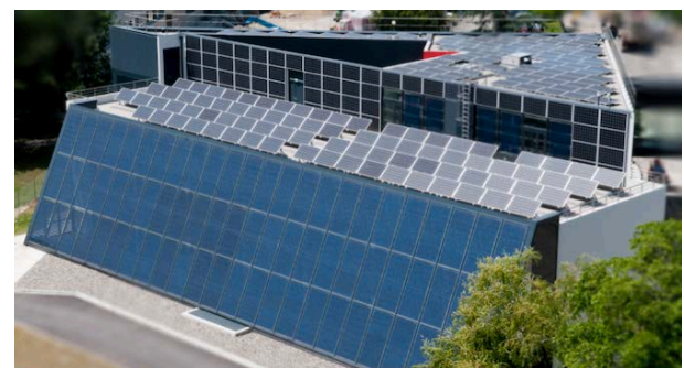
Figure 1: The Photovoltaic Windowed Façade and Roof of the Georges Girault Building
