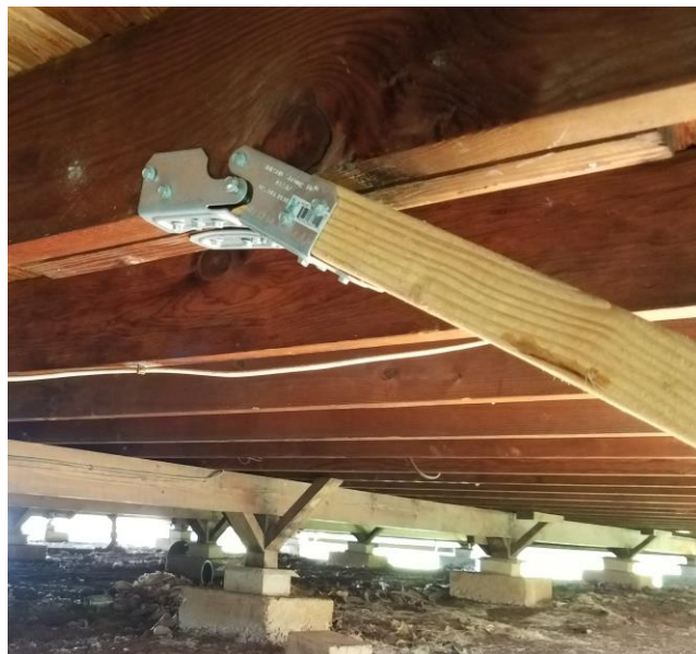
Figure 16: Two Knee-Brace Stabilizers, KBS1Z, connecting an interior brace to a floor joist.
